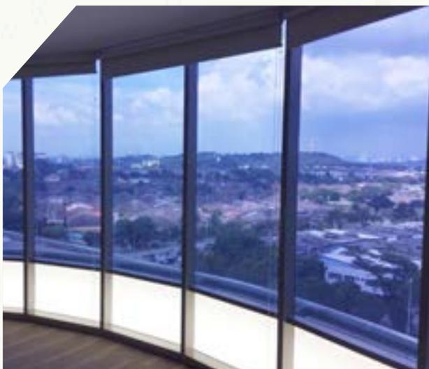
Thermal film for windows – Situated on the 8th floor with 75sqm of glasses caused of a lot of heat to be trapped inside the office. An investment in thermal transparent film to cover the glass resulted in a heat reduction of 70% and an air conditioning reduction of 3°C.
